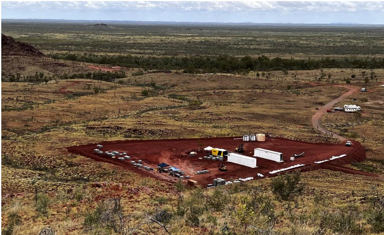
**Figure 12.** Exploration camp construction underway with levelling and compaction of 70m x 70m area in preparation for dome-sheltered core yard, accommodation, ablution block, workshop and offices. The prominent hill in the background is the western part of the Main Hill deposit. View looking southwest.
