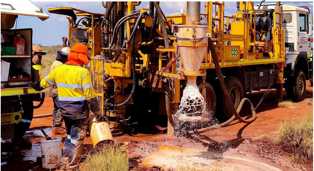
Figure 3: Aircore drilling confirms significant groundwater in hole 24KNAC004. 'Bucket test' methodology used to measure water quantities in early stages of aquifer testing.
