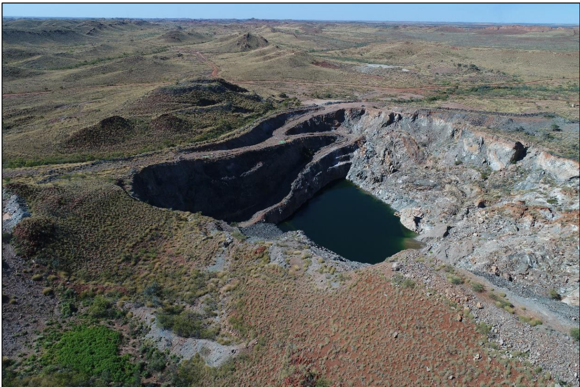
Figure 1: Drone image from the Iron Stirrup deposit area with the historical pit.
