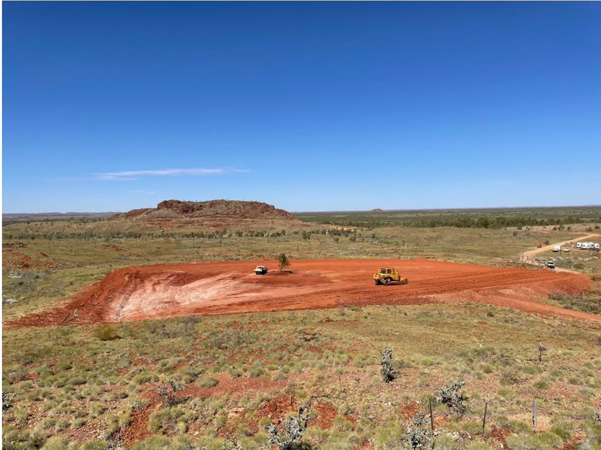
Figure 13. Exploration camp construction underway with levelling and compaction of 70m x 70m area in preparation for dome-sheltered core yard, accommodation, ablution block, workshop and offices. The prominent hill in the background is the part of the Main Hill prospect. View looking south.
